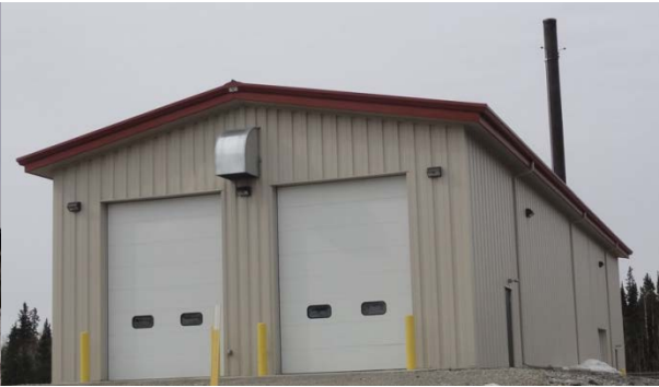
Boiler + Fuel Storage
